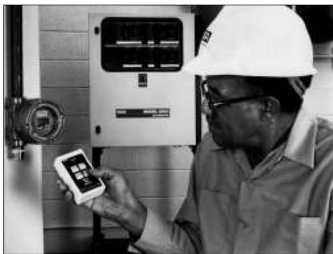
Figure 18-3. This multipoint ambient air monitor is capable of continually measuring up to five gases in as many as 24 remote locations. (Courtesy MSA.)
